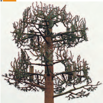
The top of a ninety-five-foot-tall wireless phone antenna made to look like a cypress tree, blending with the other cypress trees in a Metairie, Louisiana, neighborhood. (AP/Wide World Photos. Reproduced by permission.)
